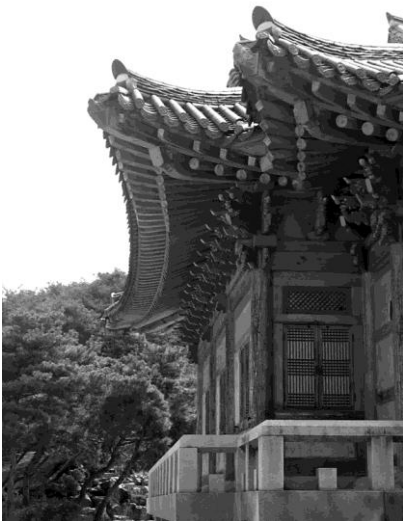
Figure 3. An example of eaves on a traditional Korean structure.
